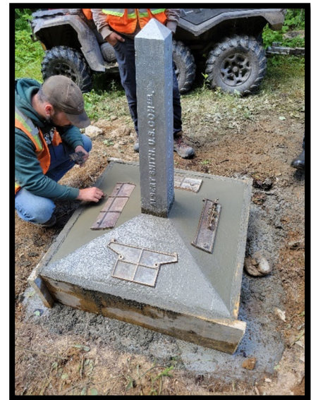
Monument identification placed during the setting of the concrete of Monument 226.
