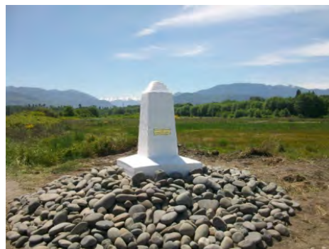
Figure 2 - Reference Mark Angeles Point after re-establishment (British Columbia/Washington)
