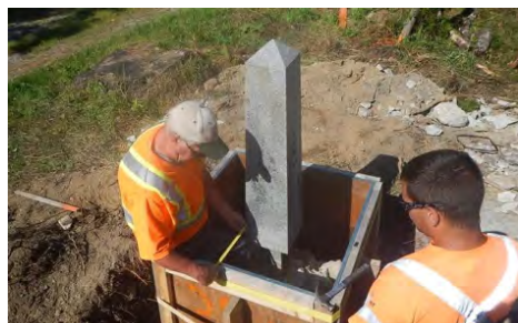
Figure 5 – A monument under construction (Quebec/New York)
