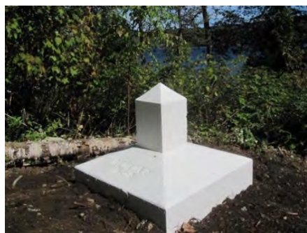
Figure 8 – Reference monument S-136 renewed (Quebec/Maine)
