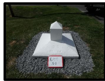
*Figure 2- RMS-54 after being graded and painted (ME/NB)*
