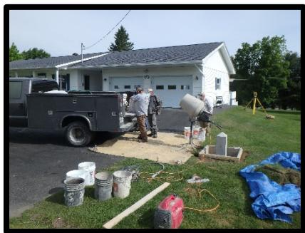
*Figure 3- Crew mixing concrete in driveway for RMS-54 (ME/NB)*
