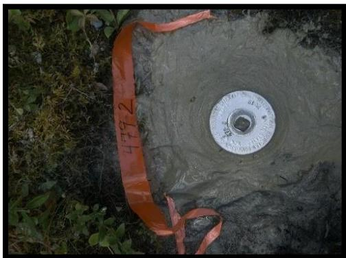
For 2019, the major maintenance work undertaken over the last few years continued in this particular section. The project saw 156 monuments renewed, 17 reestablished and 1 new monument installed. As in previous years, a new type of monument was used (an iron rock bar with an aluminum alloy cap) that should prove to be more resilient and easier to install than the previous concrete cylinders in the rugged terrain and harsh weather conditions of the Highlands.
